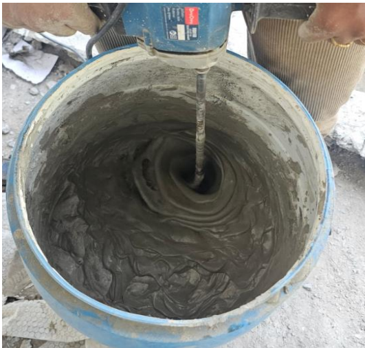
Fig no: 17 Mixing of cement, fly ash, Slaked lime and foam
