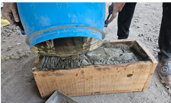
Fig no: 19 Pouring of Fresh concrete into the Mould
